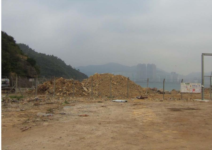
*Photo 1 –Stockpiles of the excavated materials were observed to be exposed.*
